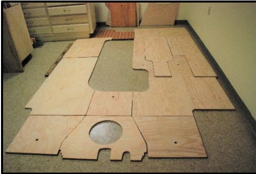
Figure 4 Layout of New Boards for Alignment
